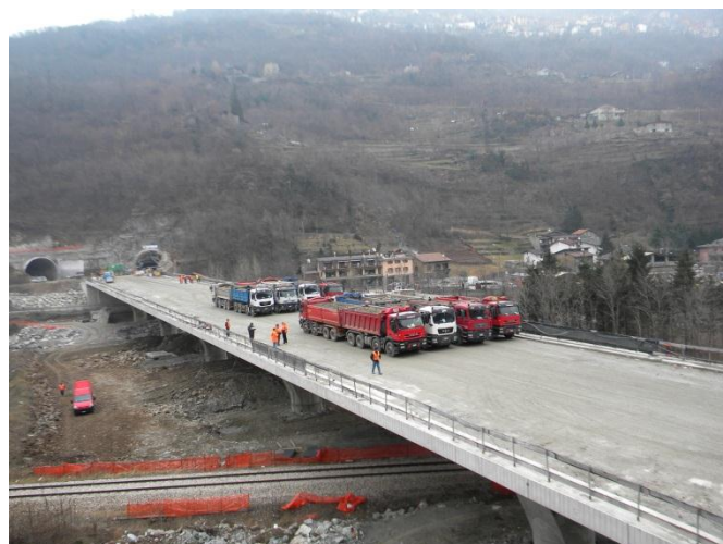
Fig. 13 – Asymmetrical load testing
